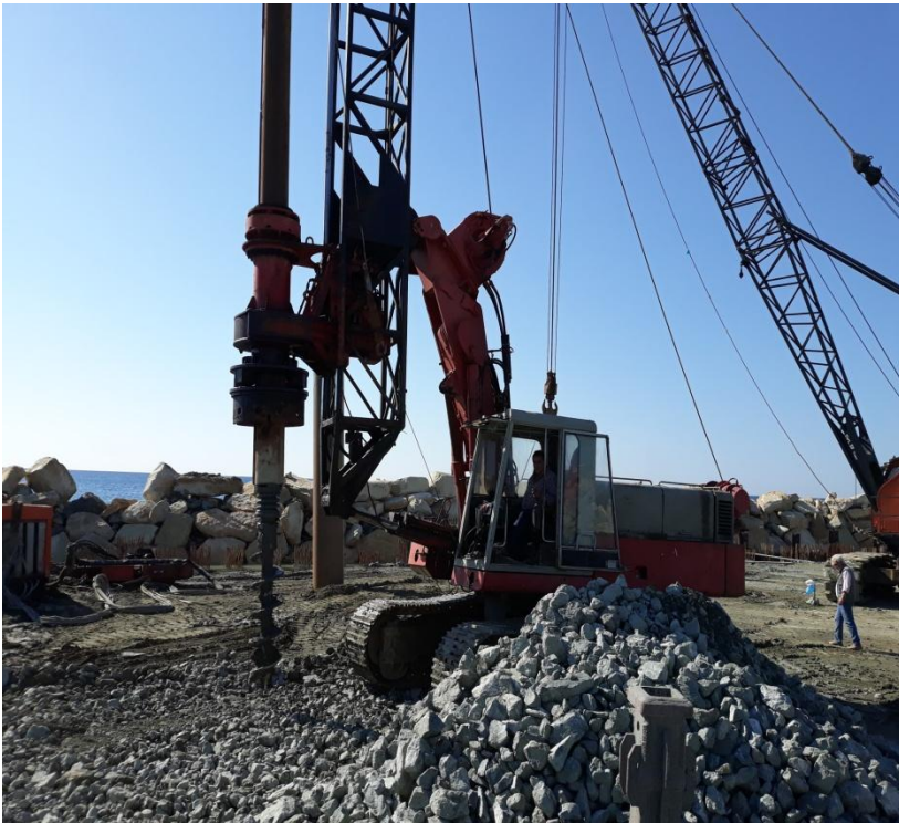
Pilling drilling machine
