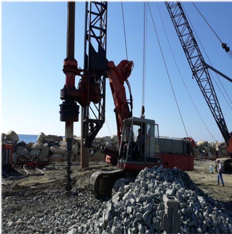
Pilling drilling machine
