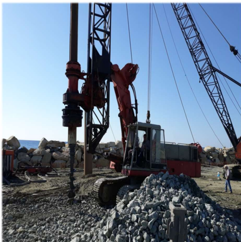
Pilling drilling machine
